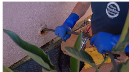
Operator two feeds the cable at the pipe.
