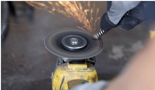
Bevel the cut edge with a grinder.
