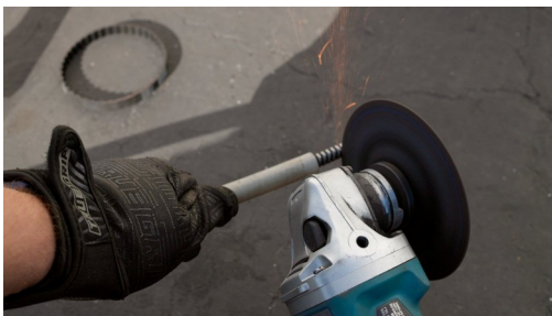
Cut off the crimped connector with a grinder or cutoff wheel.
