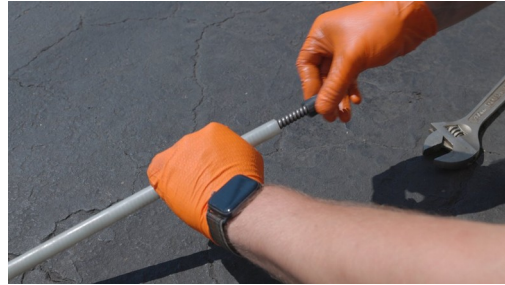
Cap removed — cable exposed.
