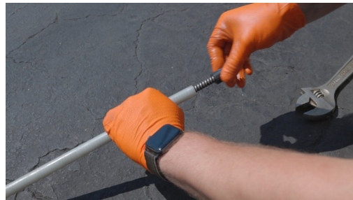
Cap removed — cable exposed.
